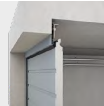
Behind The Lintel
